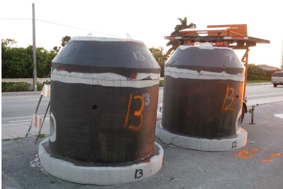
Figure 1. Coal tar epoxy on the outside of a manhole.
