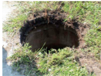
Manhole Prior to Abatement
