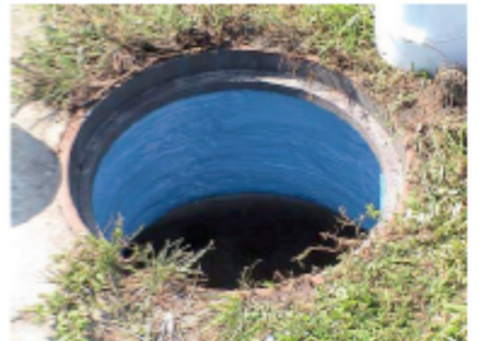
Manhole Following Abatement
