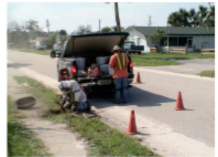
Manhole Frame / Chimney Sand-Blasted
