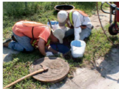
Frame & Chimney – Elastaseal® Coat
