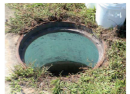
Frame & Chimney – Prime Coat
