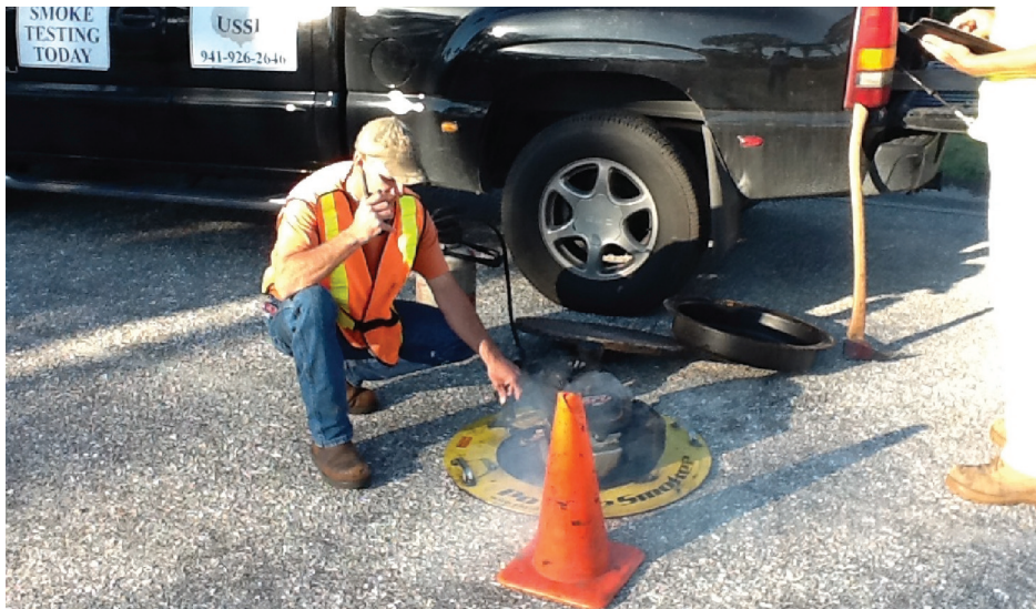
Figure 6. Smoke Test. (photo: USS1 Inc.)
