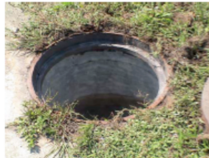
Manhole Interior Following Sand-blasting
